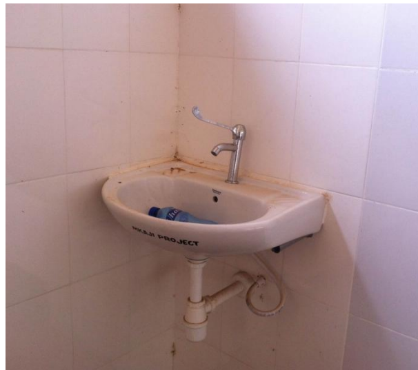
Figure 8: Hand wash sink in one of the health facility which is not in use in Dodoma region. Photo credit to Abubakari Fakhi.
